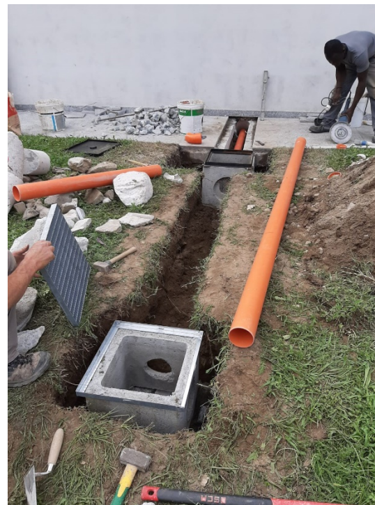
Laying of the well for exhaust fan housing and expulsion grated well
