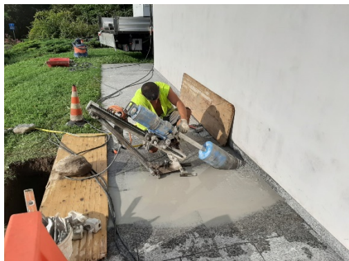
Sidewalk coring and cutting
