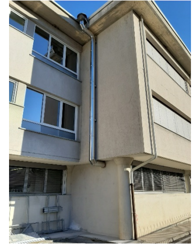
External exhaust fan with discharge beyond the eaves
