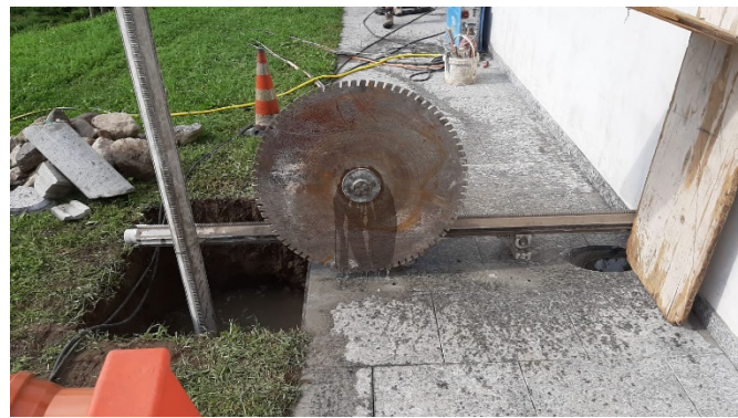
Sidewalk coring and cutting
