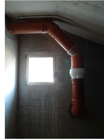
Internal exhaust fan with discharge into grated well
