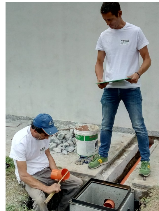
Laying of the well for exhaust fan housing and expulsion grated well
