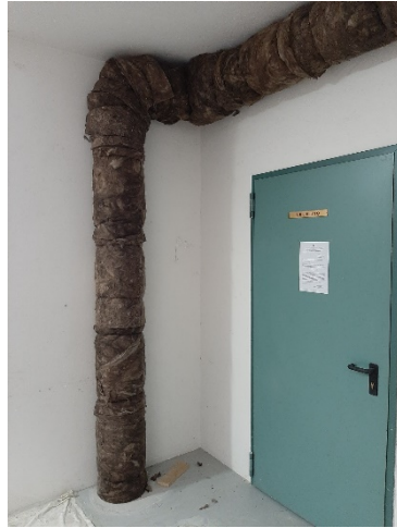
Piping acoustic insulation
